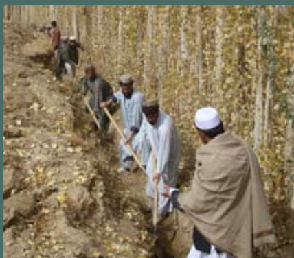
Villagers work with GPFA staff to clear a decade's worth of silt and debris from an irrigation channel.
